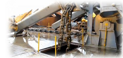
Storage in a chain locker Underside of operation deck
