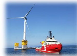
Floating wind turbine towing
